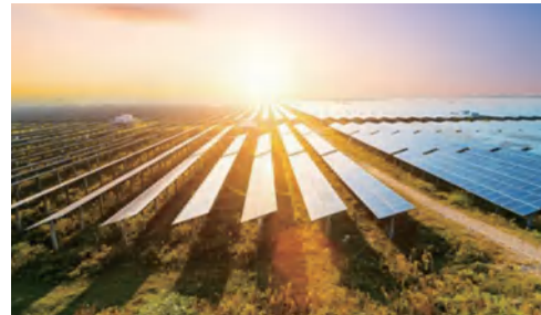
Solar Power Management
